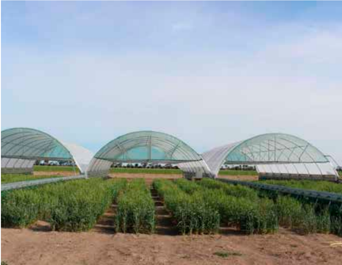
Plastic road barriers, filled with water, and steel arch frames create the skeleton for this portable rainout shelter. Photo credit Surya Kant.
